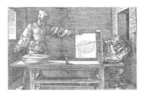
*Figure 11*. Dürer's perspectograph or instrument to draw and object in perspective
